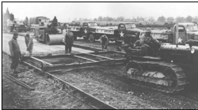
Members of an aviation engineer battalion construct a heavy bomber airfield near Eye, England, in 1943 (work commenced September 1942 – completed July 1943). US Air Force VIRIN: 130226-F-ZZ999-010
