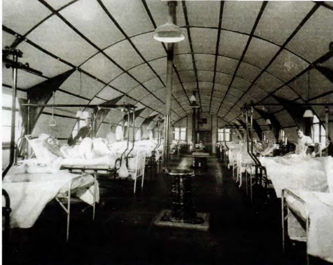
One of several orthopedic wards at 65th General Hospital. Note the small coke stove in foreground, the only source of heat. Ward floors were asphalt, kept waxed.
