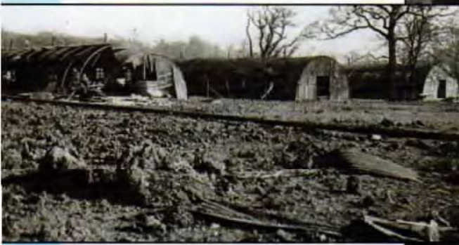
Destroyed and damaged surgical wards at 121st Station Hospital, Braintree, Essex after bombing by the Luftwaffe April 19, 1944.
