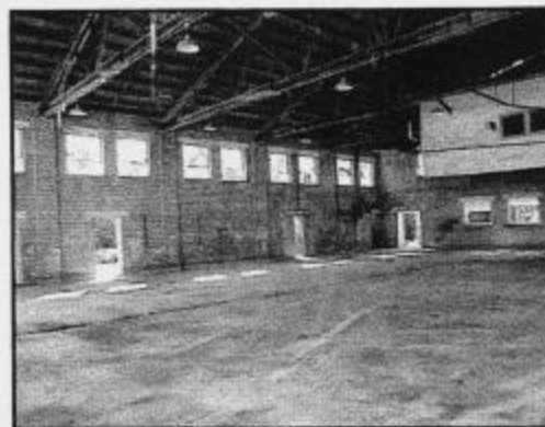
Figure 67. Interior, Hangar No. 1, 1998 (Christine Trebellas, NPS)
