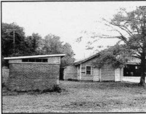
Figure 63. Locker Building & Dope Storage, Moton Field, 1997 (Christine Trebellas, NPS)
