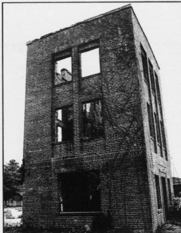
Figure 71. East face of Control Tower, Moton Field, 1997 (Christine Trebellas, NPS)
