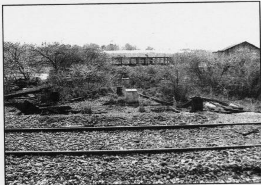
Figure 73. Remains of Chehaw, 1998 (Barbara Tagger, NPS)
