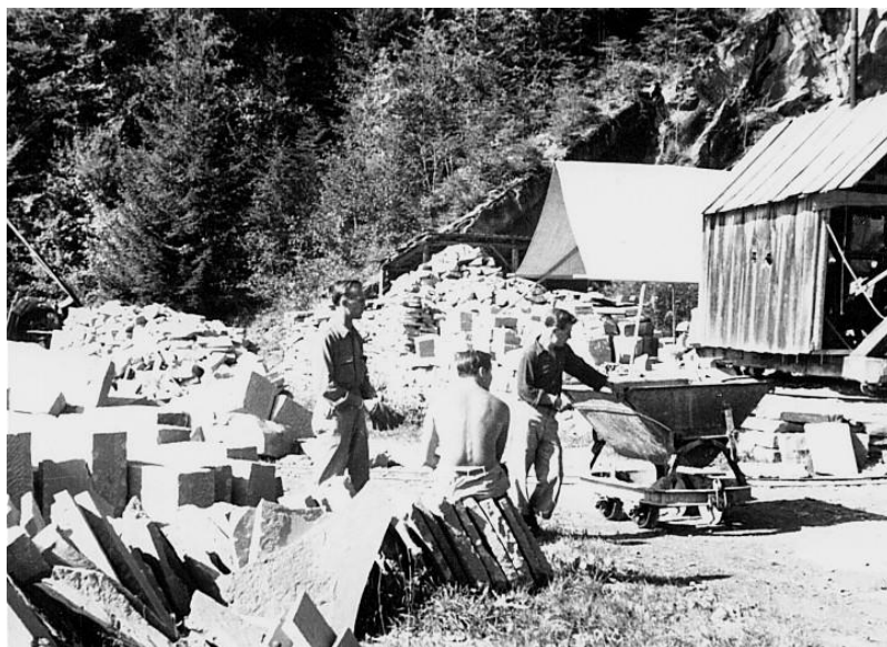
Quarrying rock at Marsens
